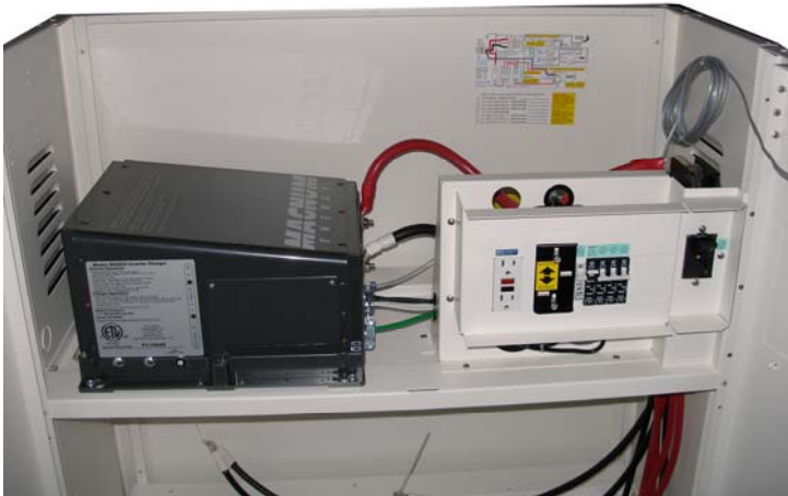
This photo shows the breaker cover installed.
